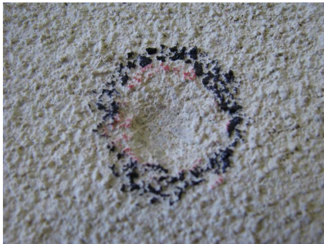
Photo 5: Typical failure when struck from front side of plate (intrusion). Hairline cracks along the outside of the indent which may not be visible in this image quality.
